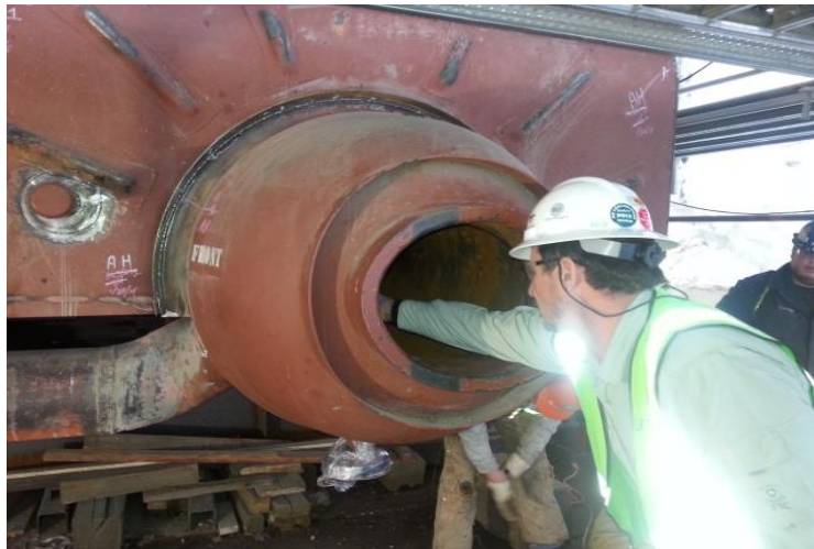
Figure 3: Steam Drum of Boiler System Liquid VCI Application
